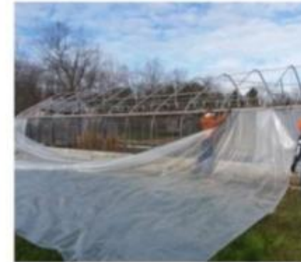
1. Remove old plastic and cut into pieces weighing approximately 50 lbs.
